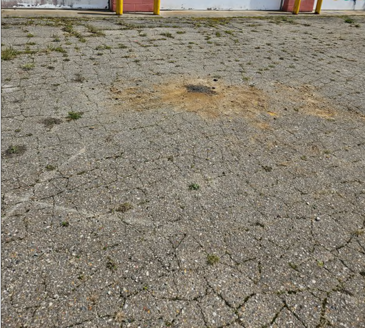
IMAGE NO. 2: Existing asphalt pavement East of proposed Farmer's Market
